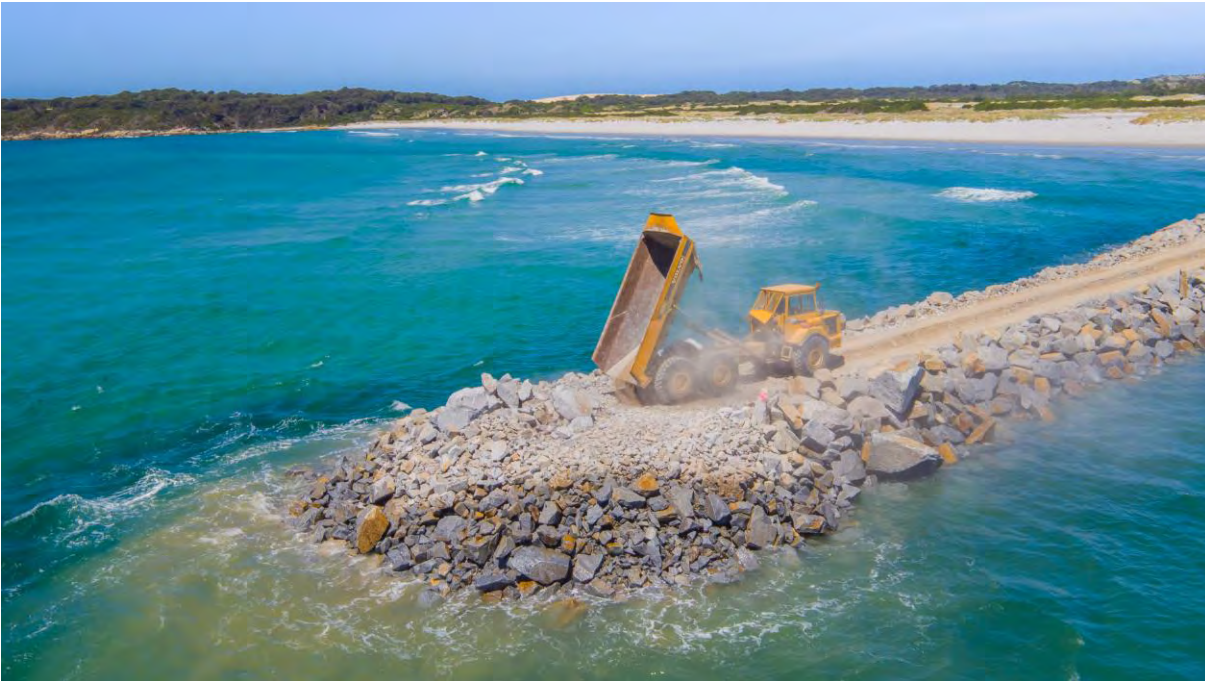
Photo 2 Example of Rock Breakwater Construction (St Helens)
