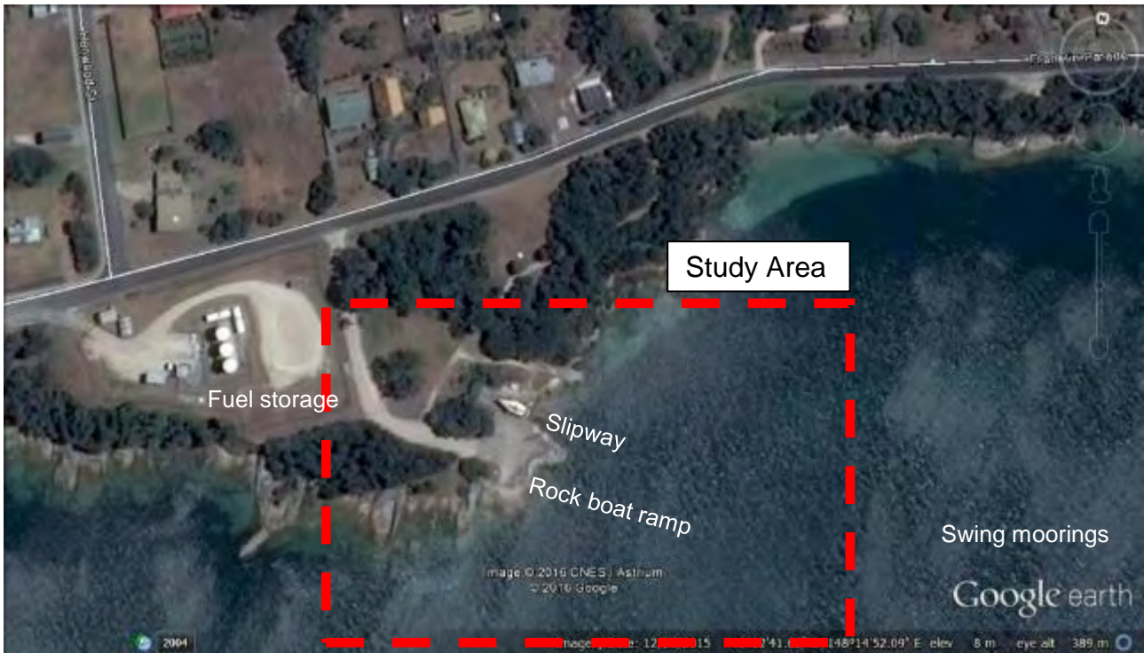
Figure 6 Lady Barron Slipway
