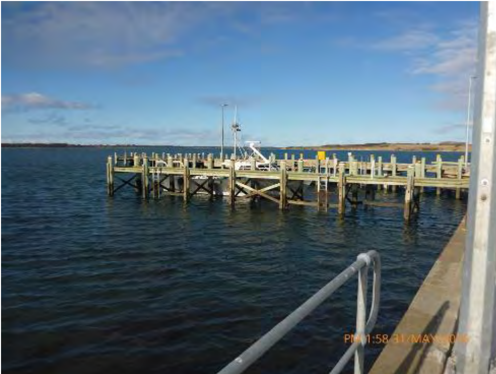
Photo 6 Port layup jetties
