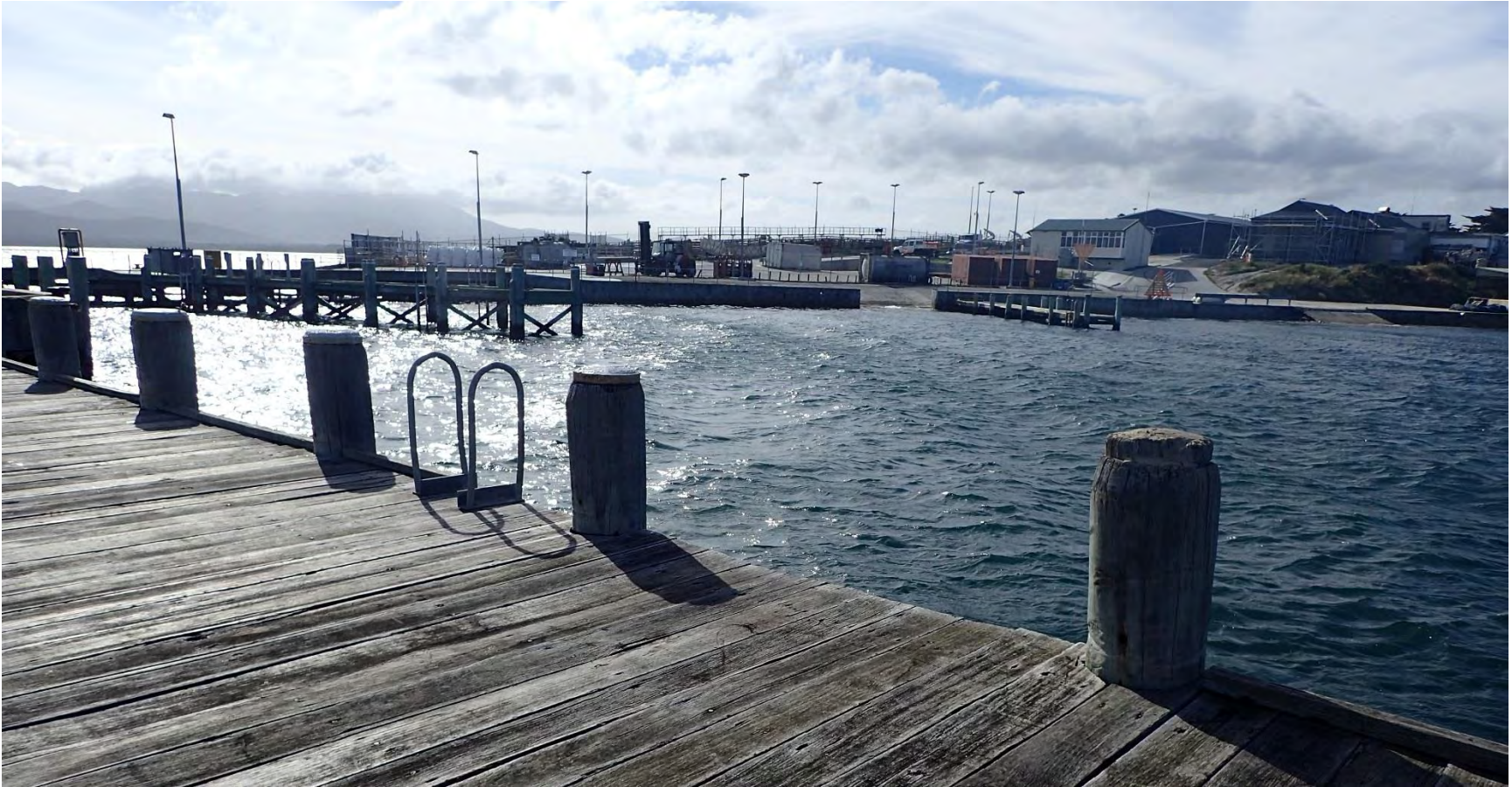
Figure 31 Photo of the shoreward facing aspect from the main jetty at Lady Barron Wharf.
