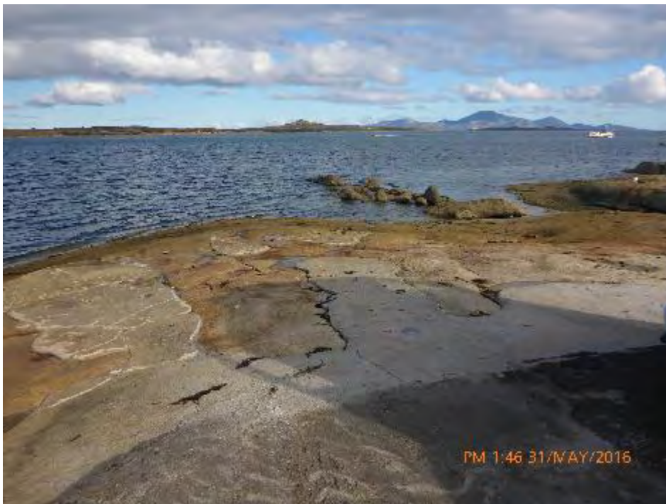
Photo 1 Existing slipway & natural rock ramp
