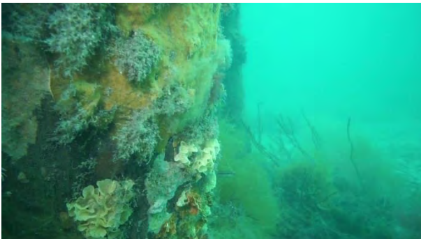
c) Piles have been colonized by a range of organisms including bryozoa, sponges, ascidians and macroalgae.
